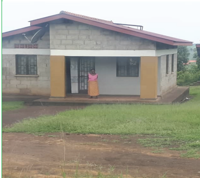
Figure 11: Some of the houses constructed for the PAPs
